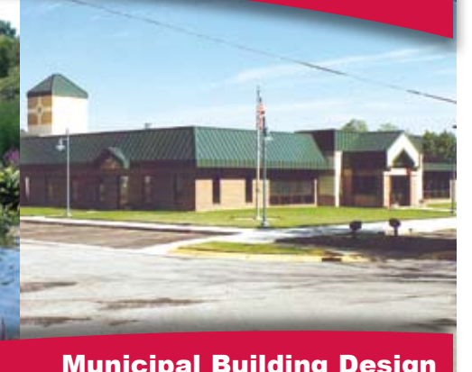
Municipal Building Design
